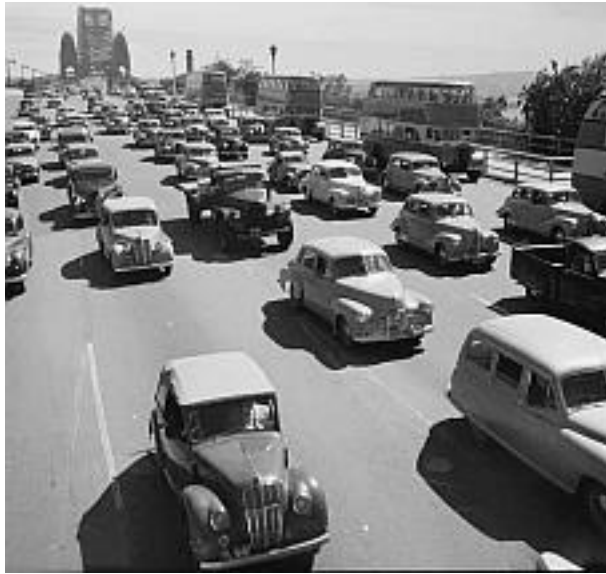
Traffic on Sydney Harbour Bridge. Photo taken around 1950.
